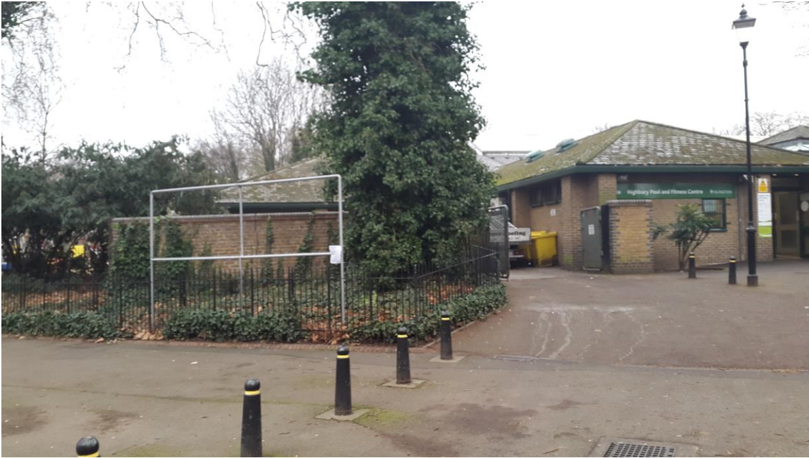
Image 2: View of front (south) elevation
